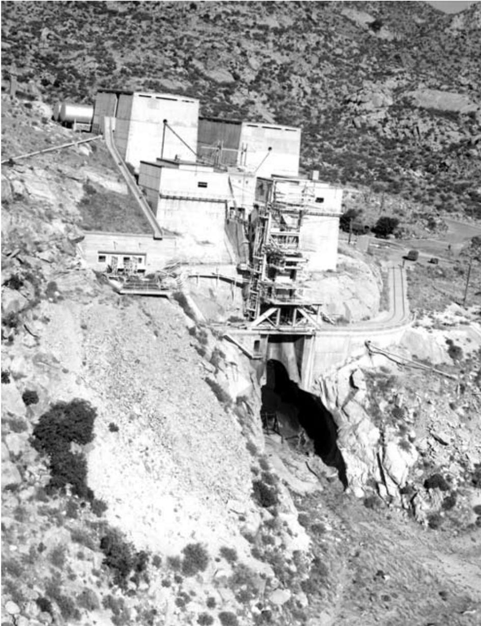
**Aerial view of the 500K static test stand west of the El Paso gate. Most people mistake it for some sort of mining structure. The pump house on the left was burned out during a wildfire that burned down the mountain from above.**
