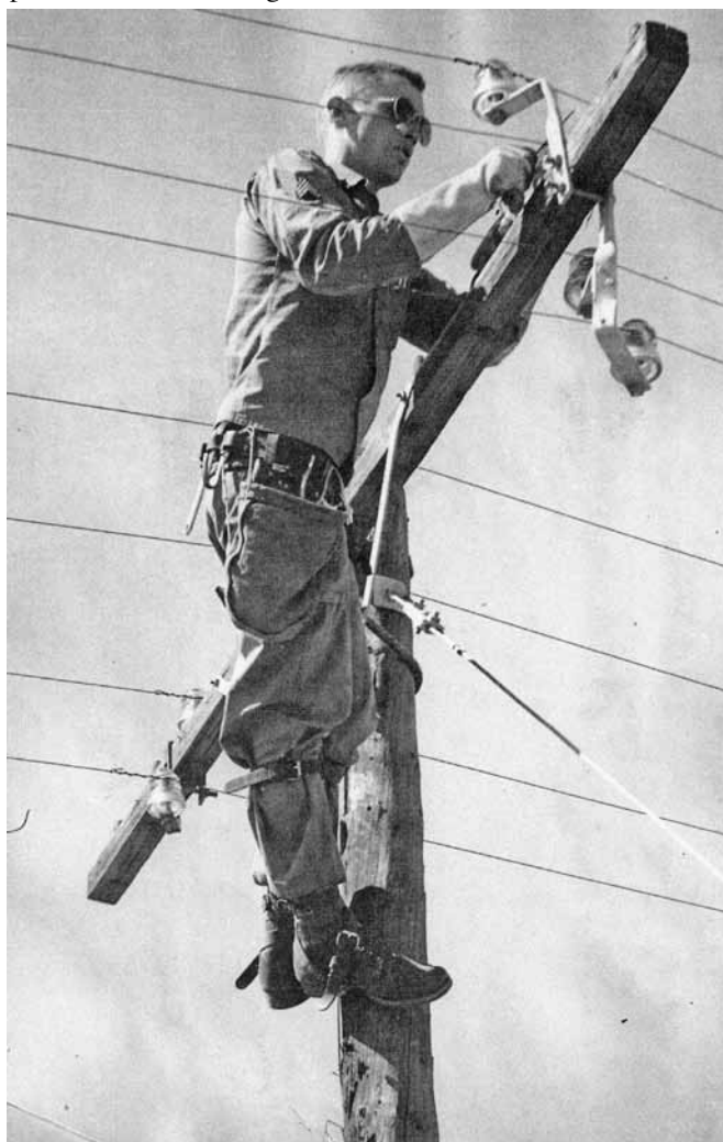
Sergeant Johnny Lay up a pole tying in open wire communication lines at White Sands in 1952.
