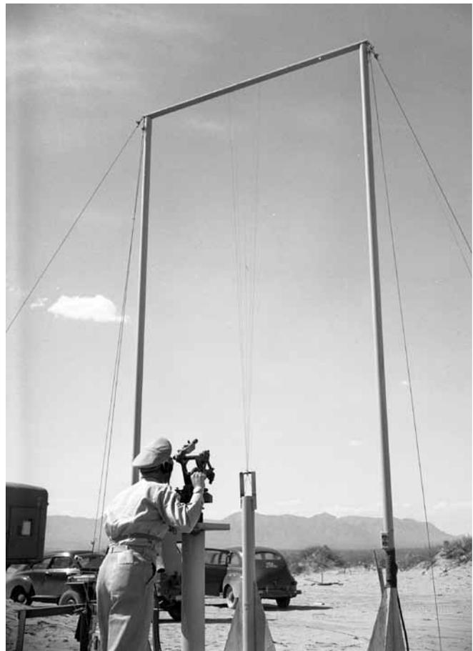
*The skyscreen system was developed after the two V-2 mishaps in May 1947 - one crashing just northeast of Alamogordo and, two weeks later, one crashing just outside of Juarez. The system used several sites perpendicular to each other. A viewer would watch the missile/rocket launch and flight through a fixed scope and he could tell if it was veering left or right. If there was an anomaly, he could radio controllers to cut the vehicle's propulsion system.*
