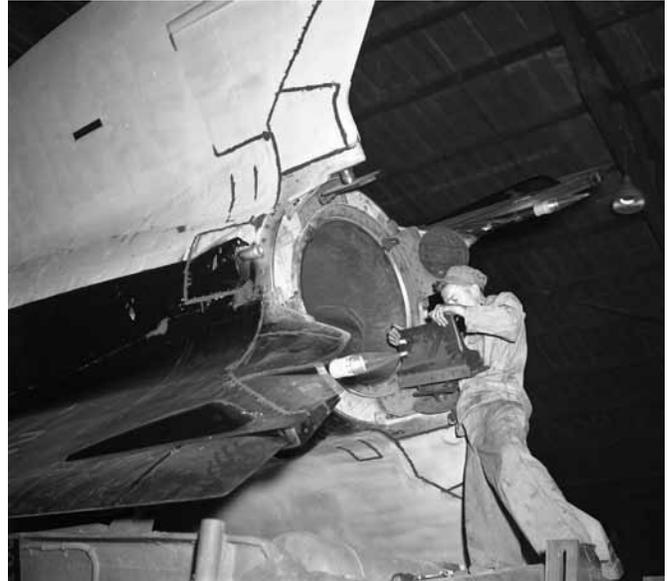
*The carbon steering vanes being attached to a V-2.*
