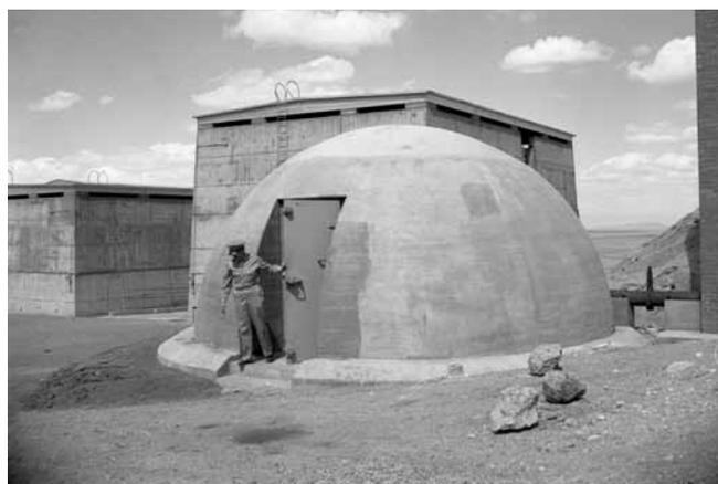
*The top photo is the spillway to drain liquid propellant away from the personnel and equipment in the event of an accident. This photo is the emergency escape bunker from the control room which is 60 feet below inside the mountain. A metal ladder inside a small shaft connects to the bunker.*
