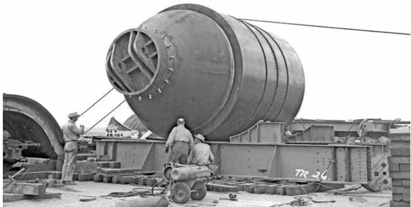
*Since Jumbo was essentially a cylinder, it was relatively easy to roll it off the railcar and onto the bed of the special trailer used to move it Trinity Site.*
