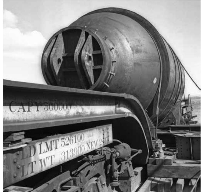
*Jumbo still on its railroad car after arriving at Pope siding. There was only one railcar in America at the time capable to carrying Jumbo's mass. Also, because of its weight and size it took a circuitous route to New Mexico to avoid some bridges and tunnels.*
