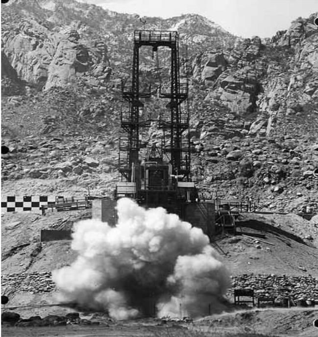
*The test of just the power system for a Corporal missile in the 100K Test Stand at a later date. An outrigger had to be added to accommodate the system. Other motors tested here included the Air Force's Bomarc and the sustainer for the Nike Ajax. The checker board structure to the left is the blockhouse. WSMR Museum Archive.*
