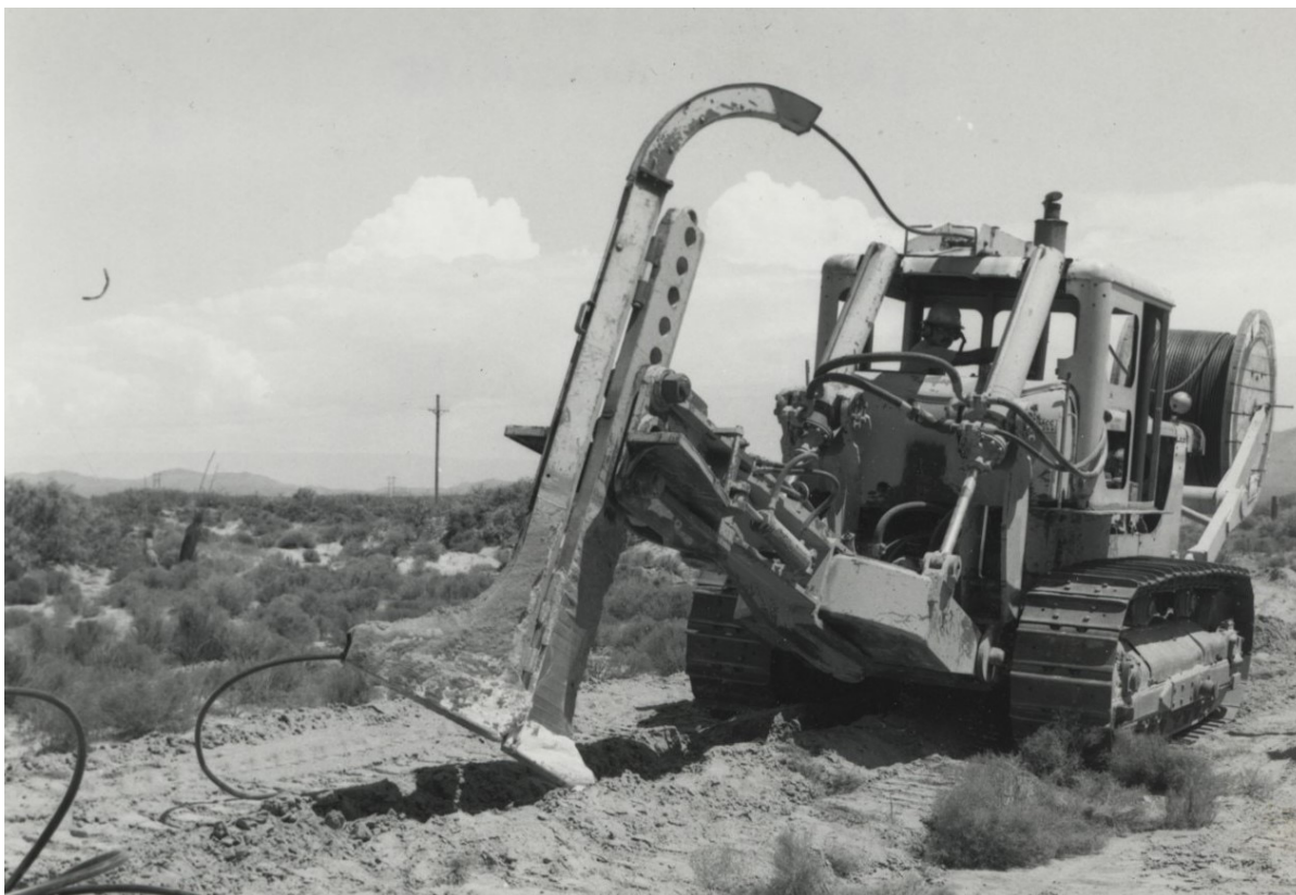
Figure 24. Cable trenching equipment laying new cable, circa 1970 ( courtesy WSMR Museum Archives ).
