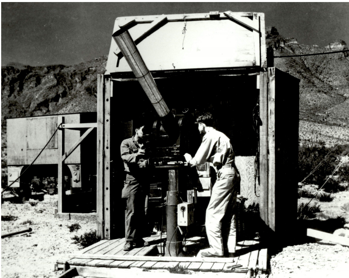
Figure 27. Early use of Askania Cinetheodolite at WSPG, circa 1945 ( Bellinger Collection, WSMR Museum Archives ).
