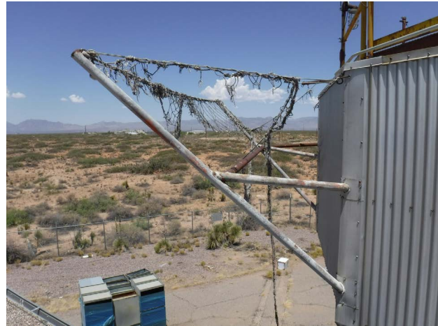
Figure 82. Property 23641, pole framework for safety net around top of tower, view to the northwest.
