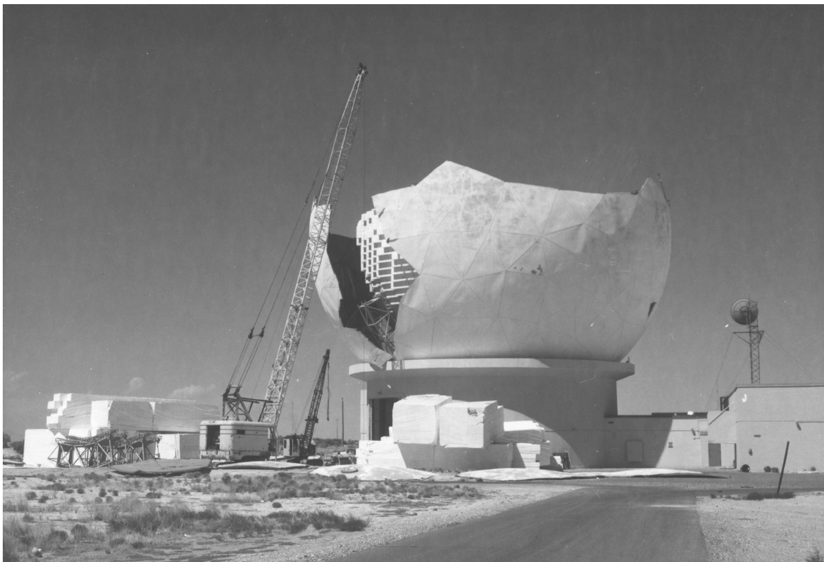
Figure 37. ZAR receiver antenna and radome under construction at LC-38 in 1960 (photo courtesy WSMR Museum Archives).
