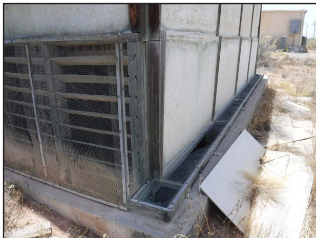
Figure 258. Property 24065, east and north elevations and vents along foundation, view to the southwest ( left ); drain into collection basin along west side of tower, view to the west ( right ).
