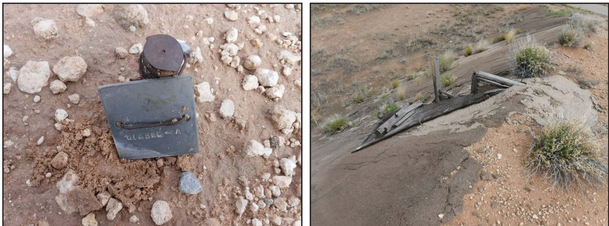
Figure 214. Patriot Pad and Revetment, “WIEBEL-A” datum atop earthen berm, plan view ( left ); wood framework incorporated into berm, view to the north ( right ).
