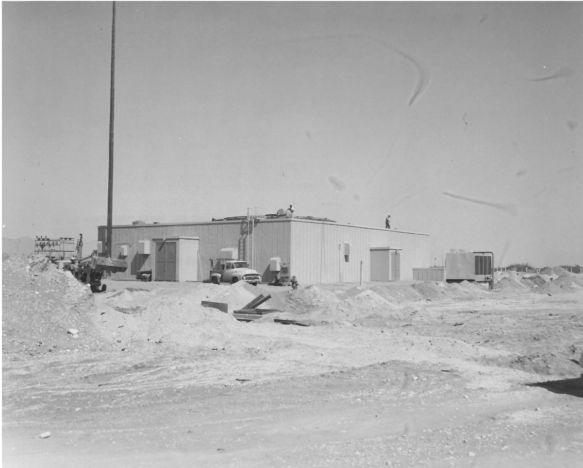
Figure 96. Property 23640 in 1960 soon after it was completed, view of south and east elevations. The terne metal shielding on the exterior is visible ( US Army photograph ).
