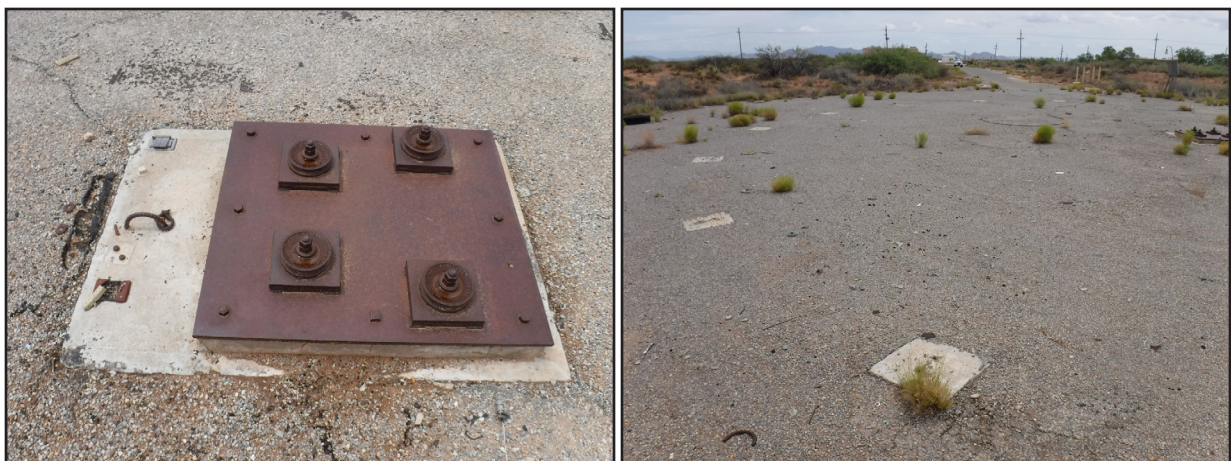
Figure 340. VEE Balloon Inflation Area, view of center slab with "sheaves," plan view ( left ); tiedown footers along north side, view to the east ( right ).
