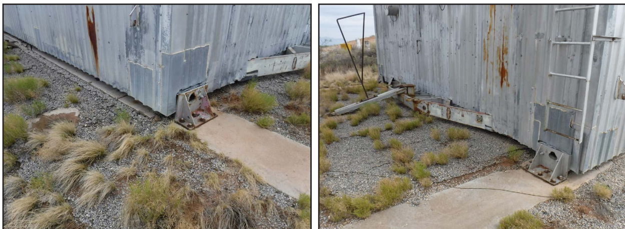
Figure 217. Travel stop at base of Patriot Conditioning Shelter rails, plan view ( left ); travel stops and hitch assembly, view to the north ( right ).
