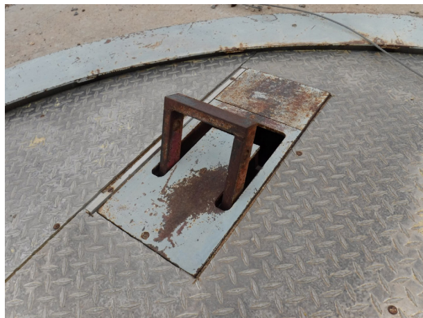
Figure 385. Detail of hinged tiedown bracket on turntable, plan view.
