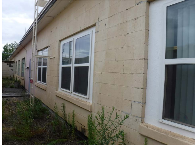
Figure 150. Property 23626, replacement windows along north elevation of CMU wing, view to the southeast.
