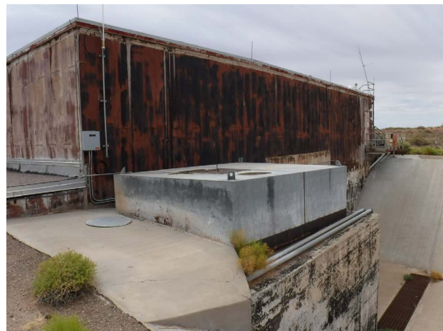
Figure 139. Property 24072, steel plate box covering on top of west elevation block, view to the southeast.
