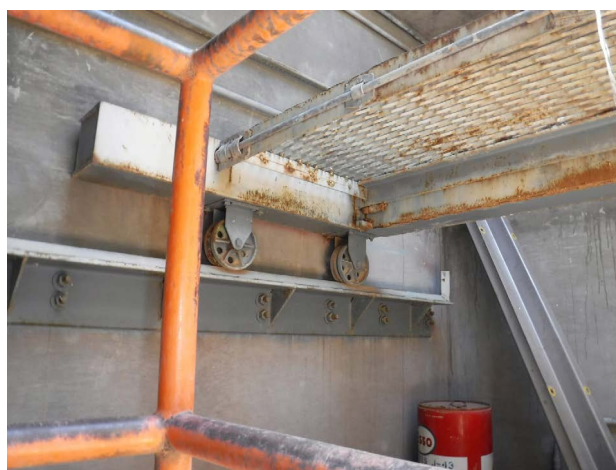
Figure 102. Property 23647, interior working platform trolley track, view to the southeast.
