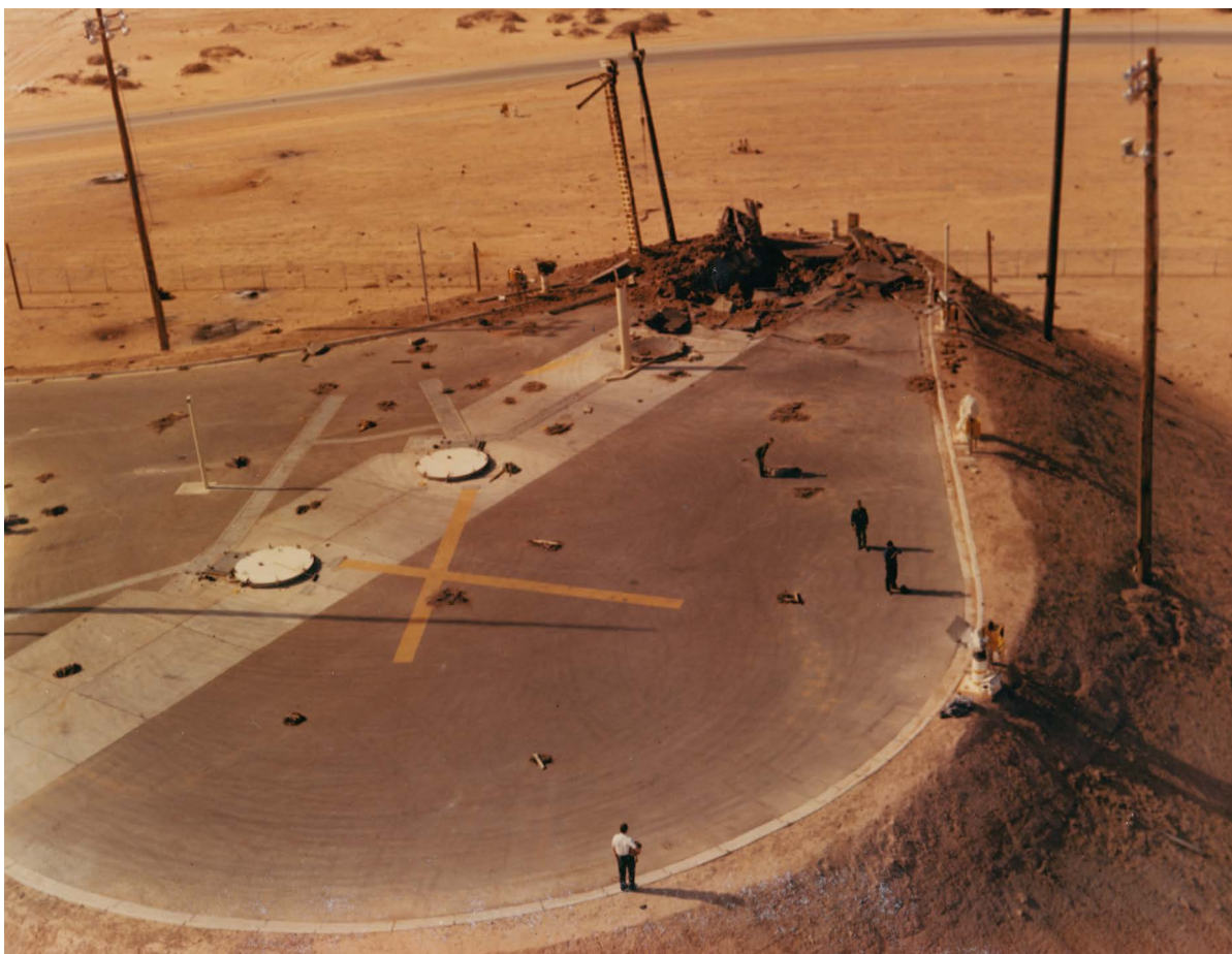
Figure 65. Overview of the damaged north launch cell at LC-50, 1965 ( photo courtesy WSMR Museum Archives ).
