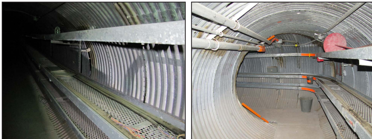
Figure 202. Cable trays and racks mounted to tunnel wall ( left ); connecting section of tunnel from Property 23683 ( right ).
