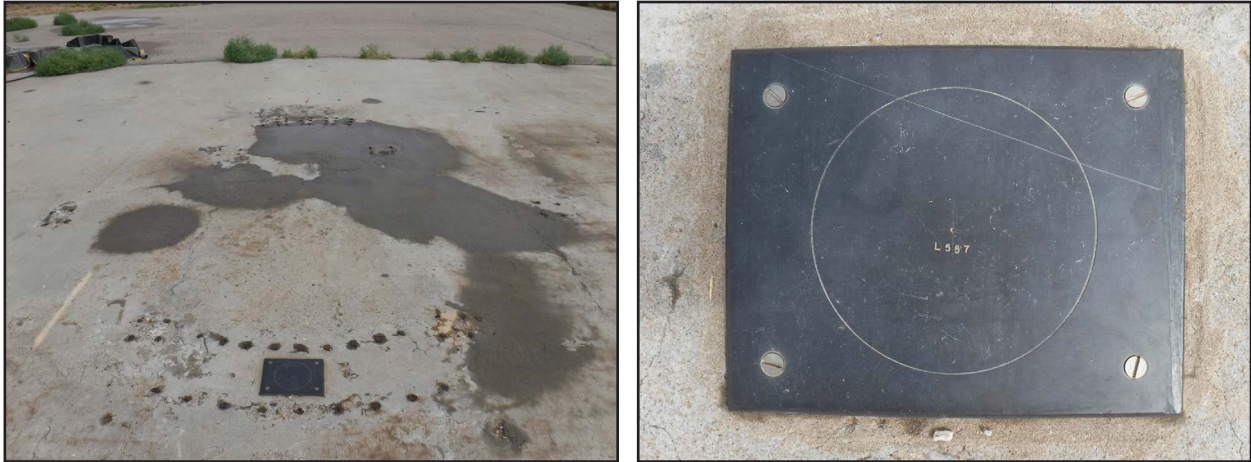
Figure 209. Patriot Launch Pad, torch-cut mounting bolts, view to the north ( left ); datum plate, plan view ( right ).
