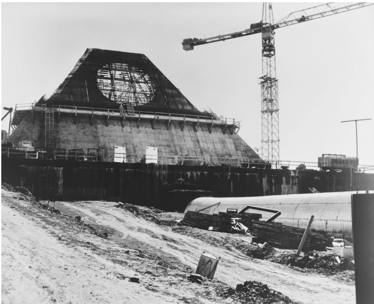
Figure 54. MSR under construction at the Stanley R. Michelson Safeguard Complex in North Dakota, circa 1973 ( public domain image ).
