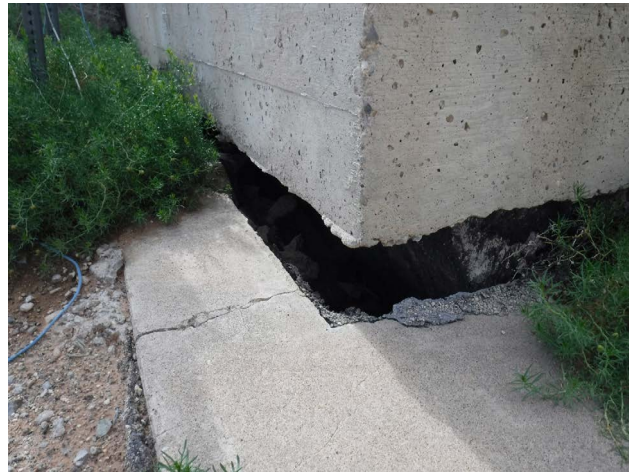
Figure 189. Property 23683, separation along south and east sides of elevated launch pad platform, view to the northwest.
