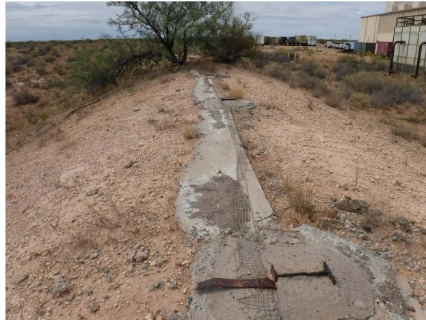
Figure 140. Property 24072, detail of concrete footer and torch-cut posts from removed clutter fence, view to the south.
