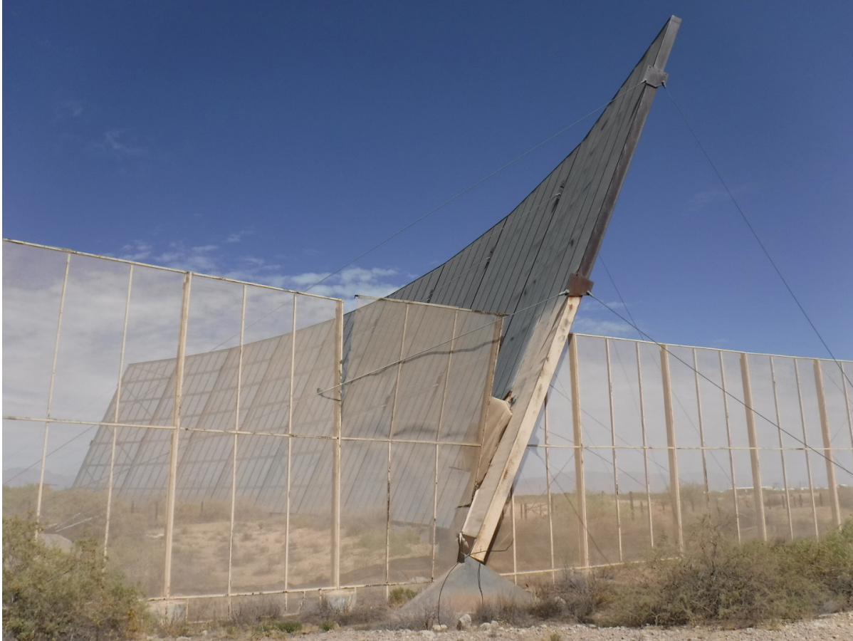
Figure 121. Property 23659, additional clutter fence panel spliced into original fence, view to the northwest.
