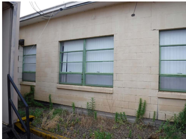
Figure 151. Property 23626, original windows along north elevation of CMU wing, view to the south.
