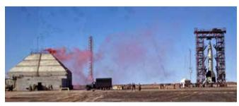
What is now Launch Complex 33 showing the blockhouse, WAC Corporal tower and V-2 gantry with a V-2 rocket in place being prepared. The red smoke warns of an imminent launch.
